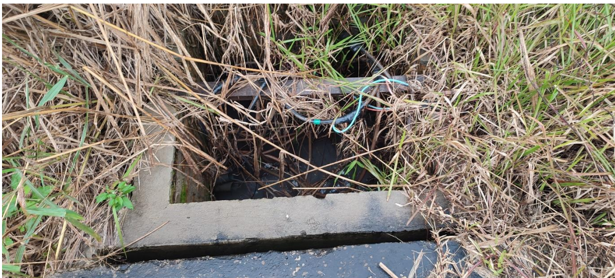
Figure 13: this is the standard access for on lot to the electricity network, cables are in water, again it looks like “make it as cheap as possible”
